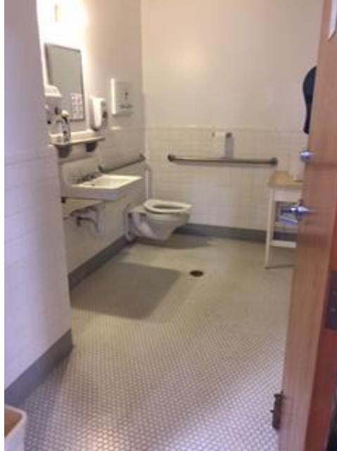
Lobby restrooms—2 of these areas
